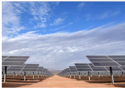
40 MW PV IN INIPAMPA PERU OWNER ENGINEER ENGIE PERU
