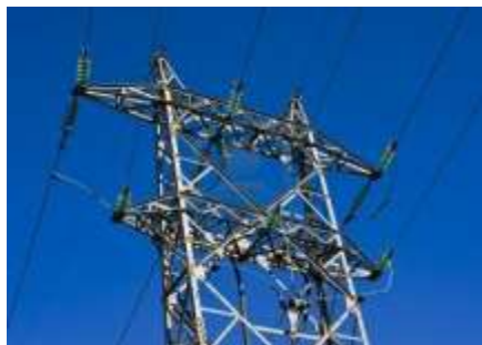
Basic and detailed engineering of evacuation electrical lines from power plants to the grid SEVERAL CLIENTS (POWER PLANTS)
