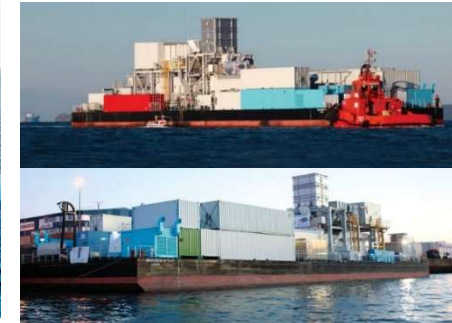
42 MW FLOATING POWER PLANT (ANGOLA) Gas turbine GE 6B UTE CUETO-SOLUCIONES
