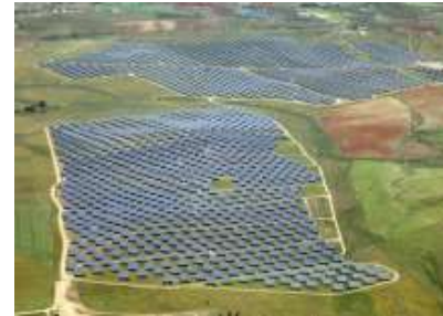
30 MW PV plant in Badajoz Extremadura ECO-ENERGIAS DEL GUADIANA
