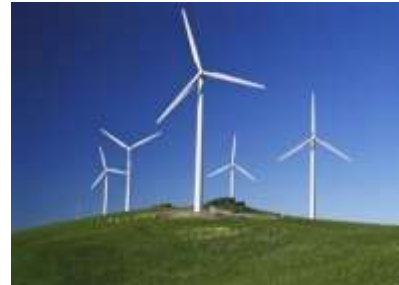
Wind farm 26 MW in Rymanow POLAND CJR WIND
