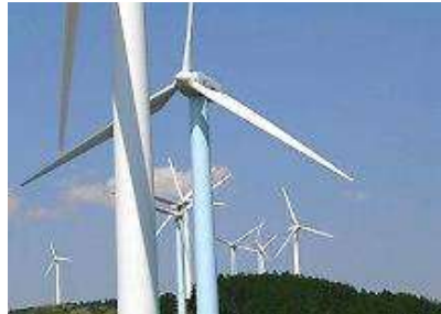
Sierra de Arcas and El Pedroso wind farms (46MW) SPAIN ENHOL
