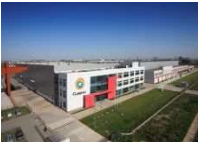
Wind Nacelles plant in Tiajin CHINA GAMESA EOLICA
