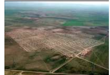
12 MW photovoltaic plant in Tinajeros Castilla - La Mancha SUNPOWER
