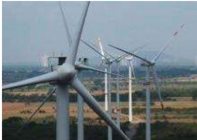
102 MW wind farm in Oaxaca MEXICO ENERGIA Y RECURSOS AMBIENTALES
